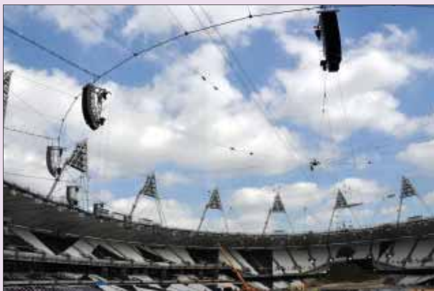
Left: 22 L-Acoustics V-DOSC hangs are suspended around the stadium via the radial cable-net system.
