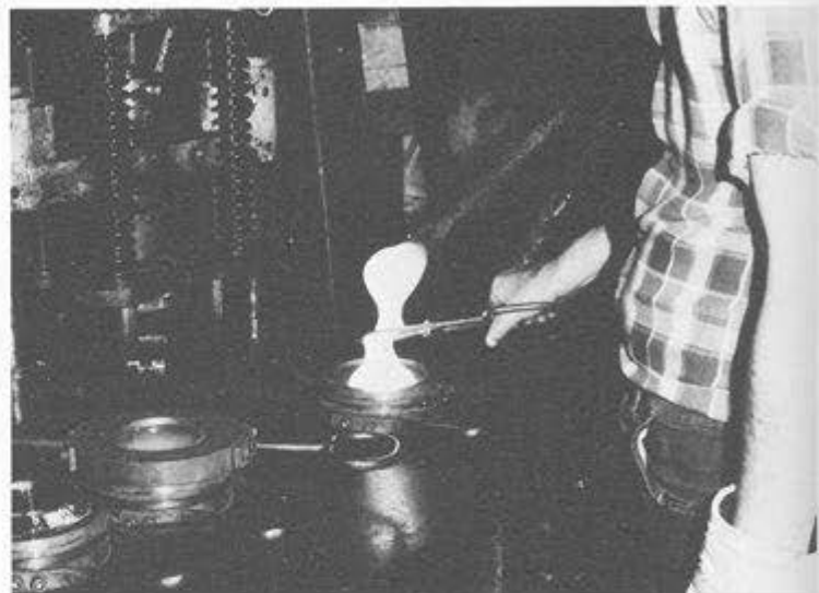
The molten glass goes into a mould.
