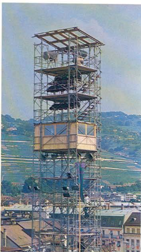
One of the four lighting towers on which were mounted a battery of 10 and 5 kW spots as well as follow spots. This one also housed the MMS control.
