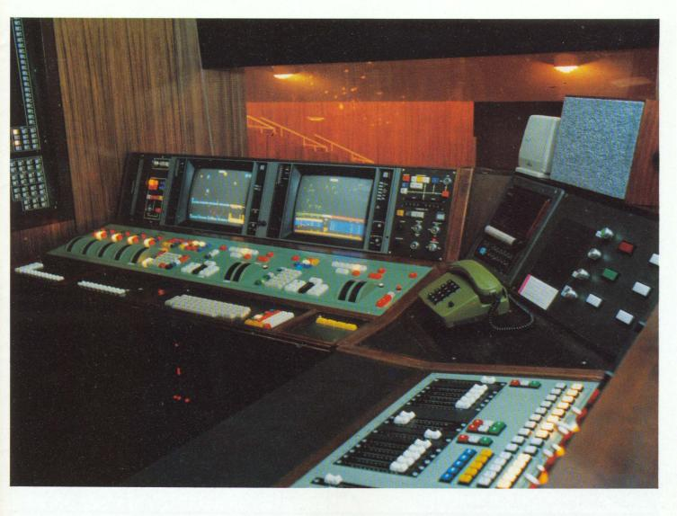
Lightboard control at Deutsche Oper, Berlin, showing horseshoe arrangement with auxiliary controls on the right-hand side and push-button mimic on the left. Close up of mimic and fault indicator system is seen below.
