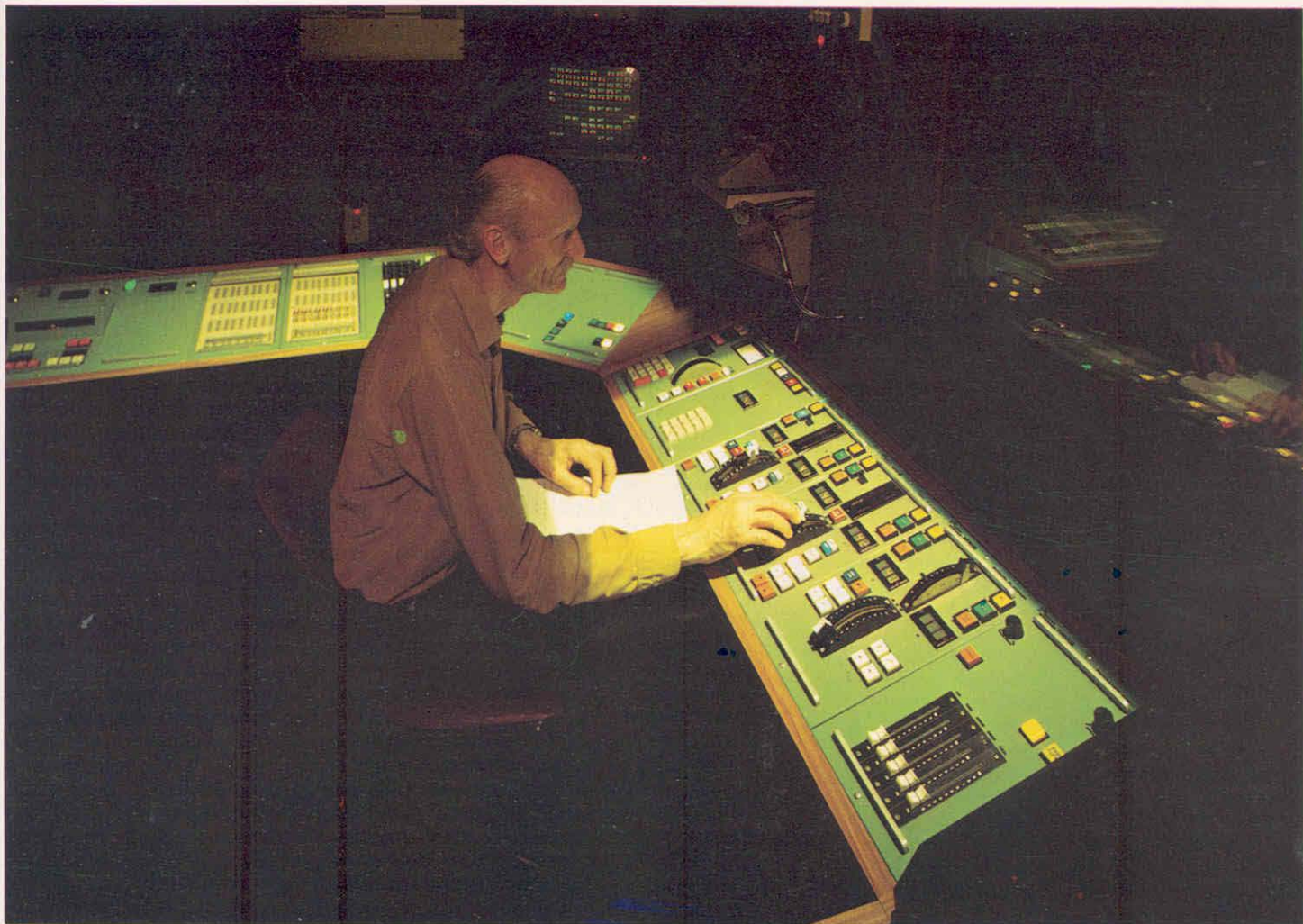
Jim Thomas, Glyndebourne's Chief Electrical Technician at the new MMS control. Opposite, another view of the control with colour Video display of channel information shown inset.
