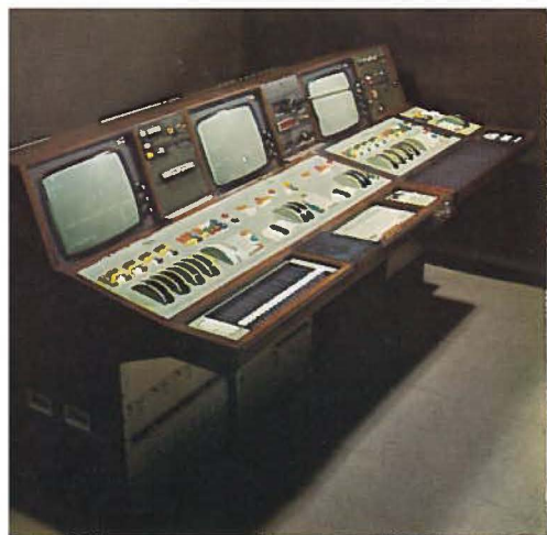
Fig. 11. Lightboard with front covers removed.
