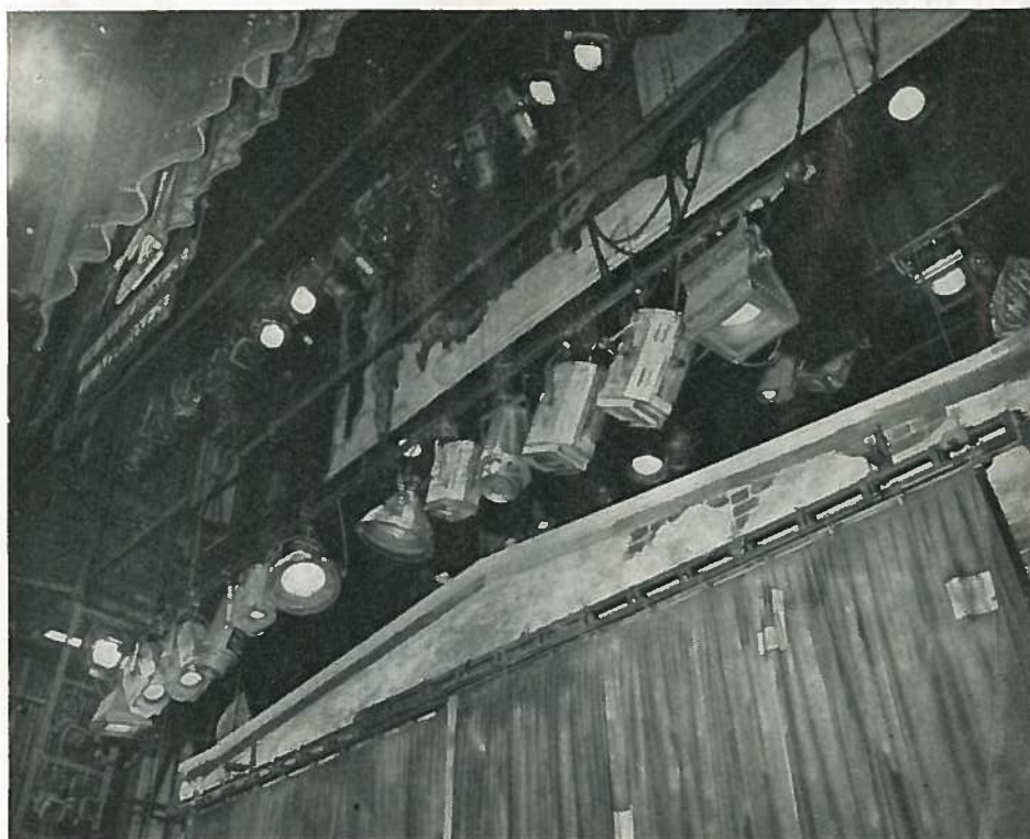
Obsolete lighting equipment is incorporated in the decor for the period backstage scenes in The Good Companions . Lanterns used include Pattern 30, 35, 43, 44, and Horizon Floods.
