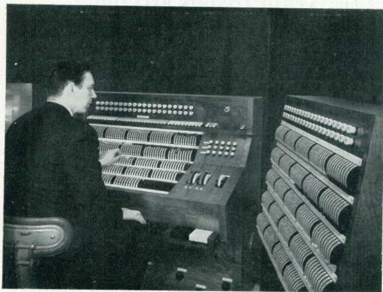
New Lighting Control room at the rear of the Grand Circle, London Palladium. Main 240-channel console on the left and movable preset wing on the right.
