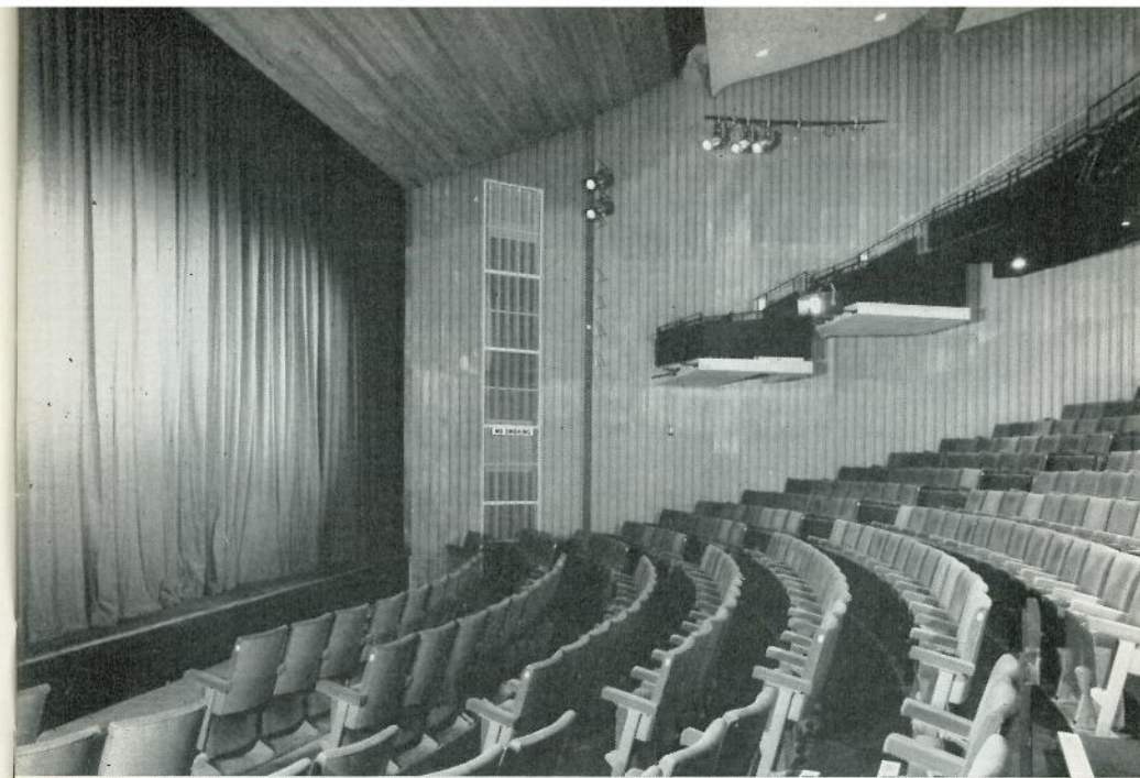
Yvonne Arnaud Theatre, Guildford. Note lighting slots in ceiling and partially occupied lighting bar and brackets on side wall.
