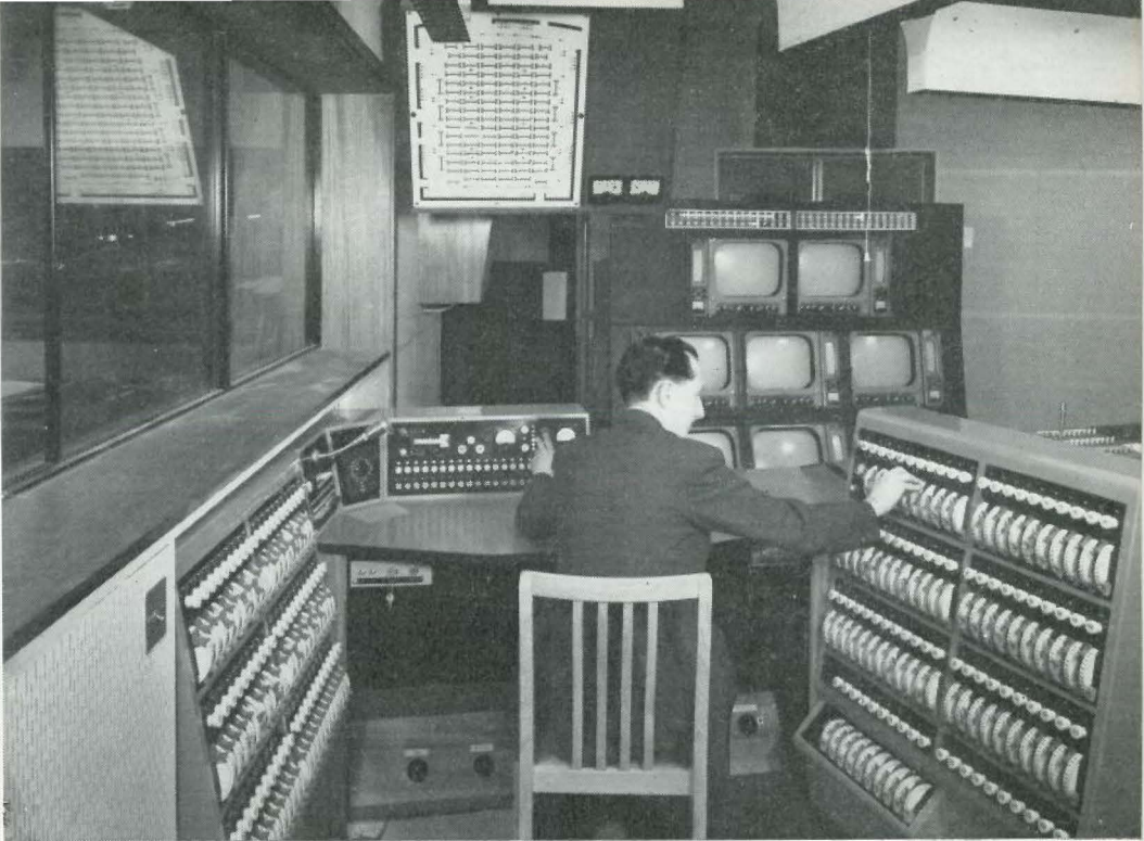
A Lighting Supervisor's station at B.B.C. Television Centre: Strand lighting control to left and right of operator with Master desk centre and Mimic diagram of studio outlets overhead.
