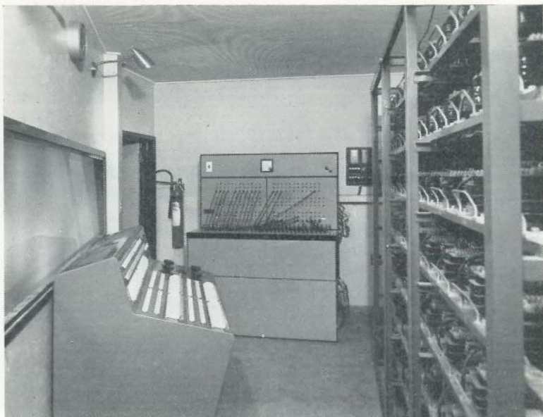
Fig. 5. Control room covers have yet to be fitted to rack—the show was more important.
