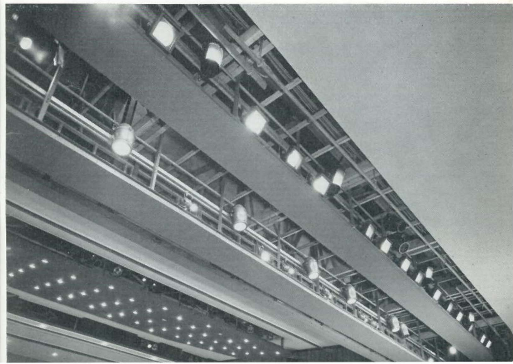
Fig. 2. Catwalks and bridges above stage. Top of cyclorama on right.
