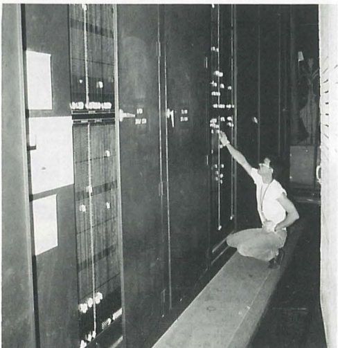
Back stage, the magnificent old Electro sliding contact patch panel. All this has come down to a key pad on current Electro systems!
