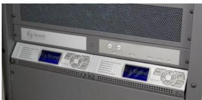
*Single or dual electronic modules control up to 144 dimmers per EC21 rack (192 dimmers for C21). Panic controls may be wired to external switches/systems as required.*
