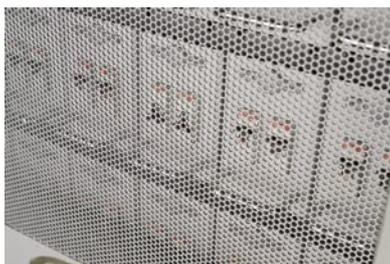
EasyView™ door assures safety and total security while allowing users easily to identify circuit-breaker trips
