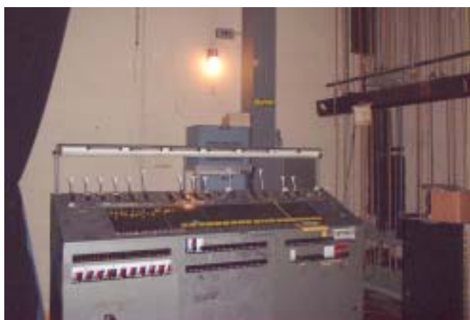
The original dimming system with its built in patch panel took up valuable wing space.
