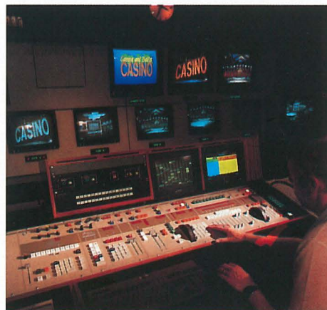
■ All Yorkshire TV's three studios are controlled by Galaxy boards. Peter said, 'We had been talking about controls here for some years. When we came to the ordering — we felt that the Galaxy was really the only one which was suitable for our needs. All the dimmers were replaced by Strand PIP dimmers.' A fourth Galaxy is used for outside broadcasts or as a Stalls control in the studio.
