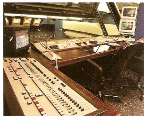
■ Galaxy 3 systems control auditorium lighting.
