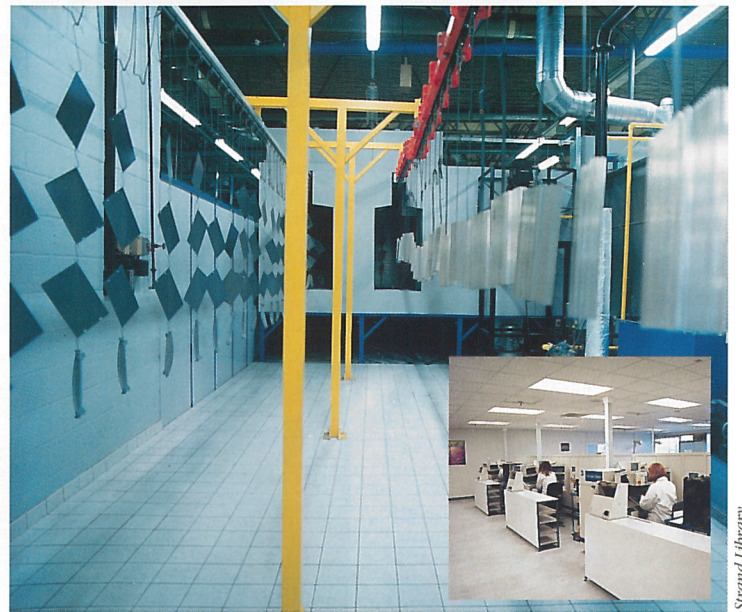
Part of the new electrostatic paint plant with the PCB facility (inset).
