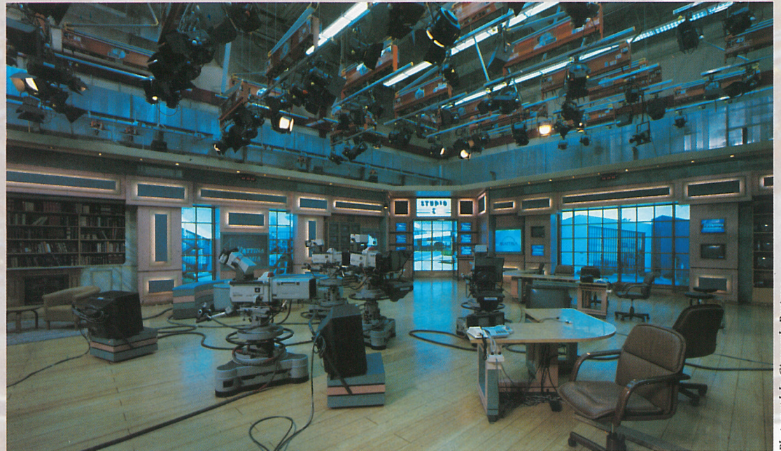
One of the nine new studios at Radiotelevisione Italiana (RAI) Rome.
