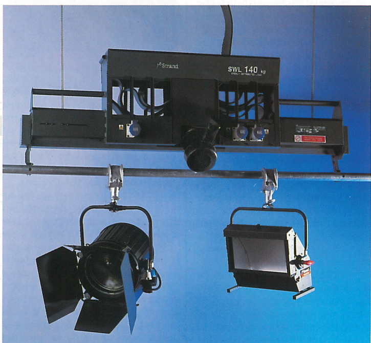
One of Strand's self climbing hoists as installed at both Ulster TV and RTM Malaysia
