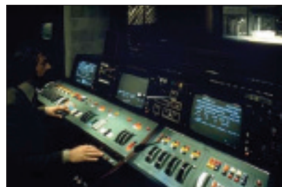
The Strand Lightboard at the National's Lyttelton Theatre. Peter Radmore is at the controls. (photo: courtesy Richard Pilbrow)
