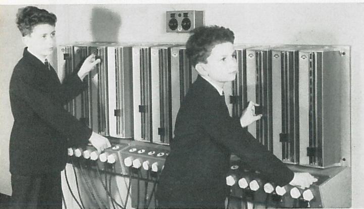
24-channel 12-dimmer switchboard made up of three Strand Junior 8's. The switching allows all circuits to be dimmed simultaneously and its use by several pupils at a time is also readily possible.
