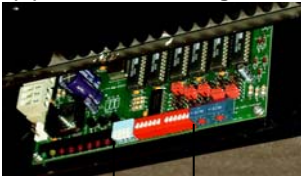
Panic and Worklight switches
