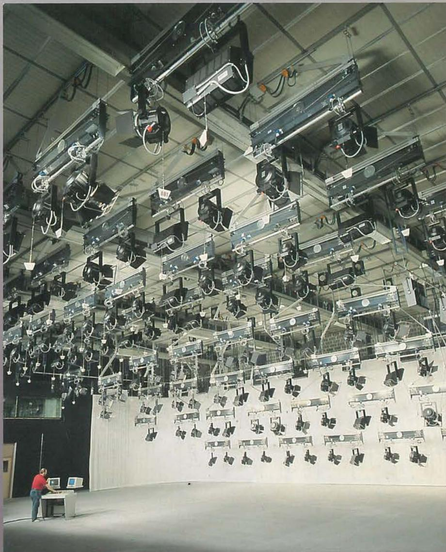
This new television studio in Hannover is probably the world's most sophisticated automated lighting facility. A studio floor control panel allows both lighting levels and positions to be adjusted to a very fine degree. Strand not only provided the PALS fixtures and control gear, but also supervised the design and complete installation.
