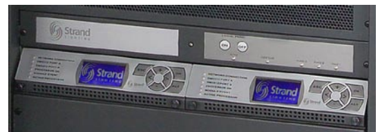
Single and Dual Electronics are available for control of up to 144 dimmers
