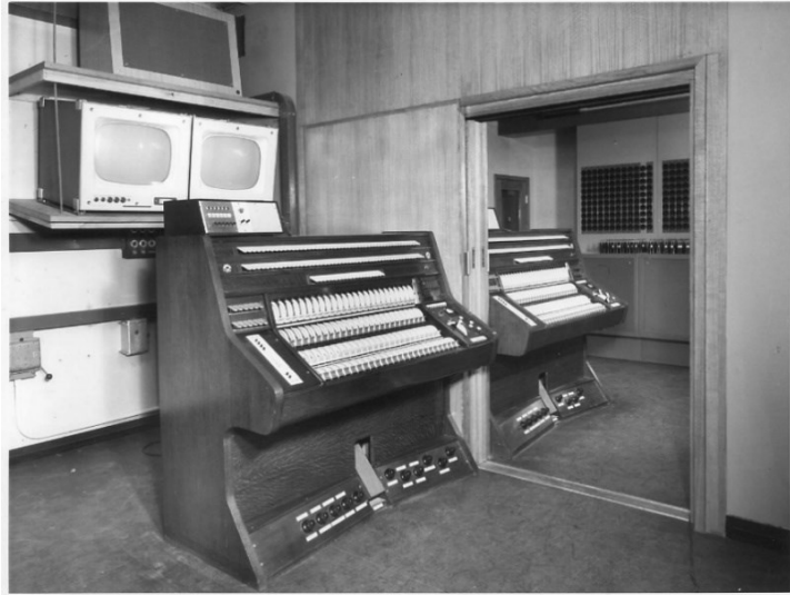
Two Strand System CD TV lighting consoles with conventional Compton hardware and memory pre-sets, in adjacent BBC Television installations, Wembley Studio 5, UK.
