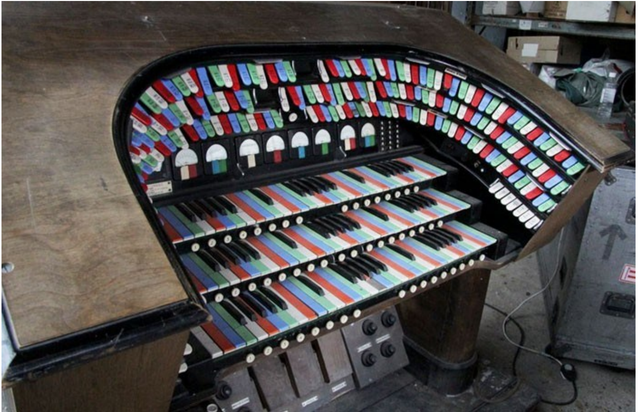
The Strand Light Console, Theatre Royal, Drury Lane. London (installed 1950; operational till 1975) with 216 independent lighting circuits across three keyboards, programmable thumb pre-set pistons, dimmer indicator dials and separate speed pedals for each manual. Each sweep would control two remote mechanical dimmer banks of the type as pictured previously. The combination setter board at the rear of the console contained 1,728 setter switches. Note vii
