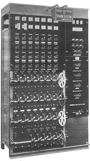
The above are two types of dead-front switch and dimmer boards. The one on the left is a 3-colour board, with 15 ampere tumbler switches, back of board colour master switches, bracket type dimmer handles, quick motion master wheels, and slow motion worm drive.
