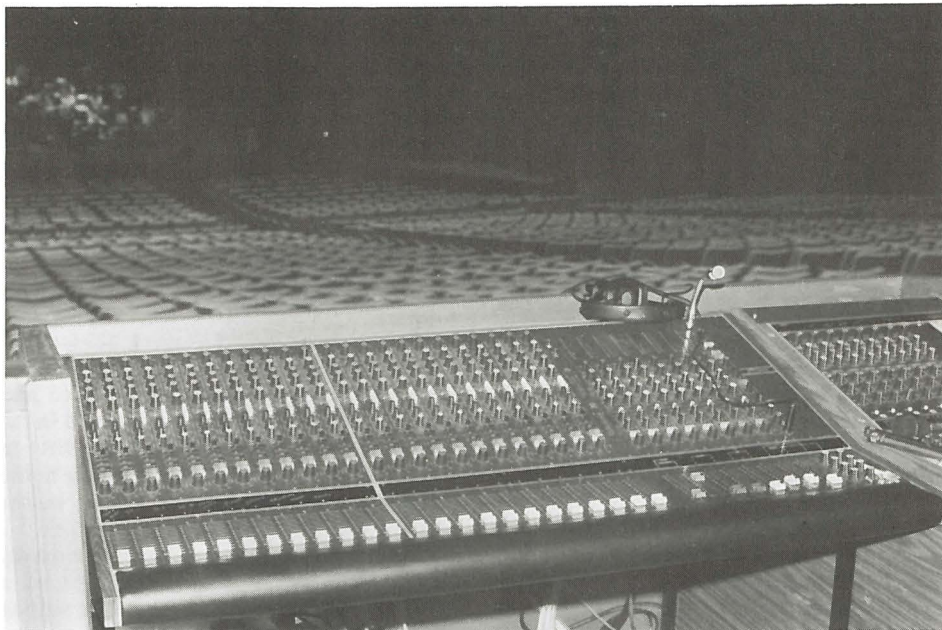
63 input, 8 group mixing desk at the rear of the stalls
