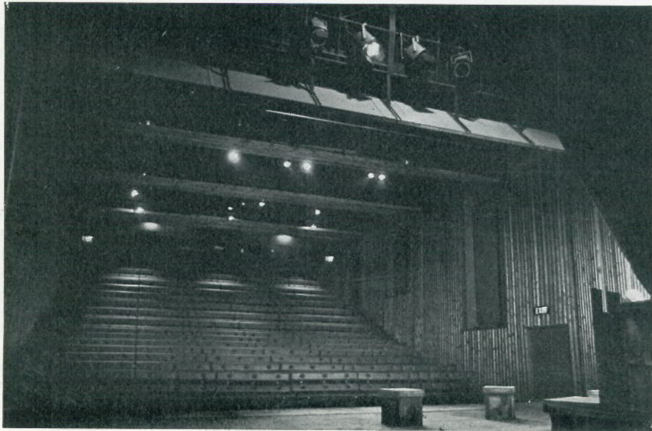
Uppingham Theatre showing (above) adjustable proscenium and (below) FOH lighting bridges behind ceiling slots. In the foreground part of the stage gantry.
