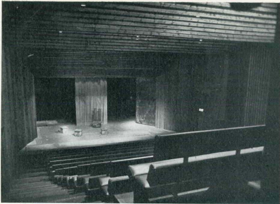
Uppingham Theatre showing (above) adjustable proscenium and (below) FOH lighting bridges behind ceiling slots. In the foreground part of the stage gantry.
