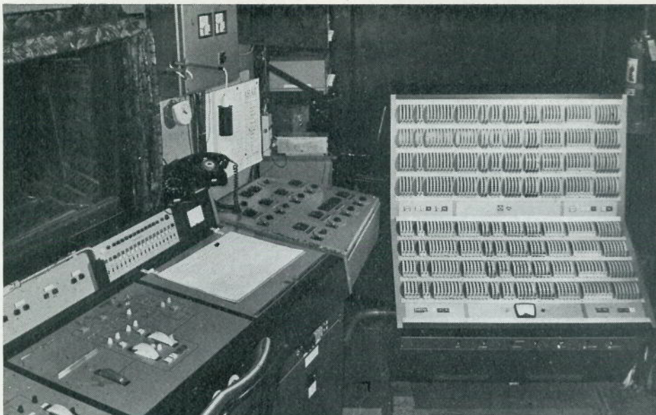
The 220 dimmer channels at the Hungarian State Opera, Budapest. On left, master desk; on right, wing housing Preset 111 of the L.P. with levers for the I.D.M. (the automatic) underneath.
