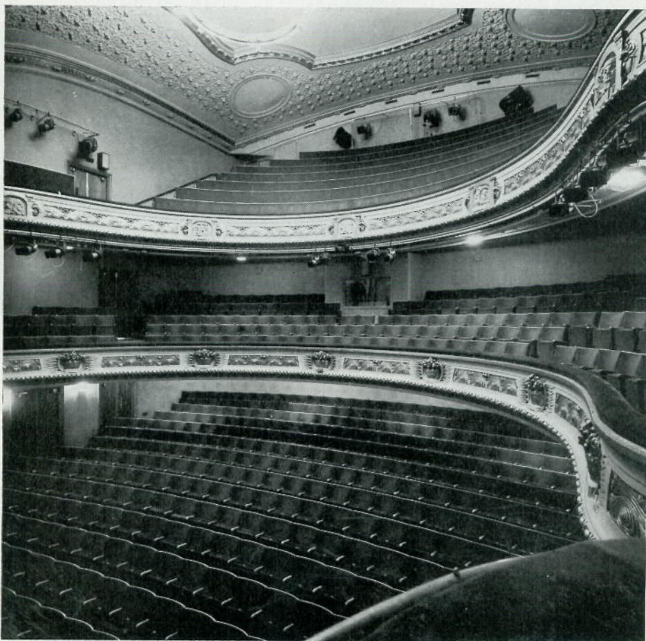
Norrköping Stadsteater, Sweden. Lighting suspension bar can be seen round the upper circle. Photo on previous page shows stage manager's observation point in the stage box.
