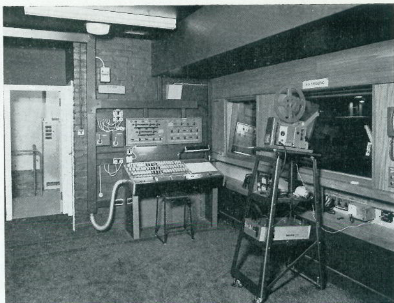
The spacious control room at Craigie which houses the 3 preset 40 channel lighting console. The dimmers are just visible in the room beyond.
