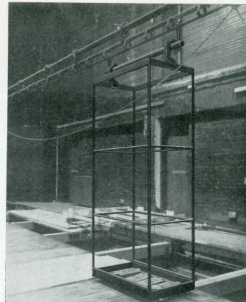
This shows the special cradle running on a heavy duty tab track for focusing and maintenance of the spot bars. Note the counter weights in the bottom of the cradle which are removed after the electrician has stepped into it.
