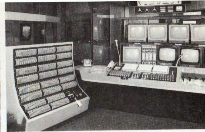
Lighting control and mimic diagram, BBC T/V Centre, Studio 6.
