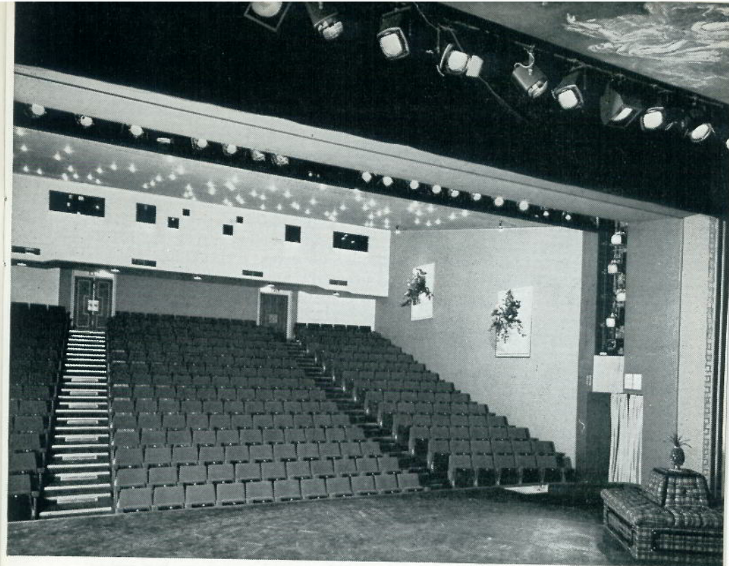
Adeline Genée Theatre. Auditorium showing No 1. Spot Bar over stage and FOH lighting slot. System SP 3-preset 2-group 60-channel (20 FOH, 40 Stage) control is housed in room above the left-hand exit.
