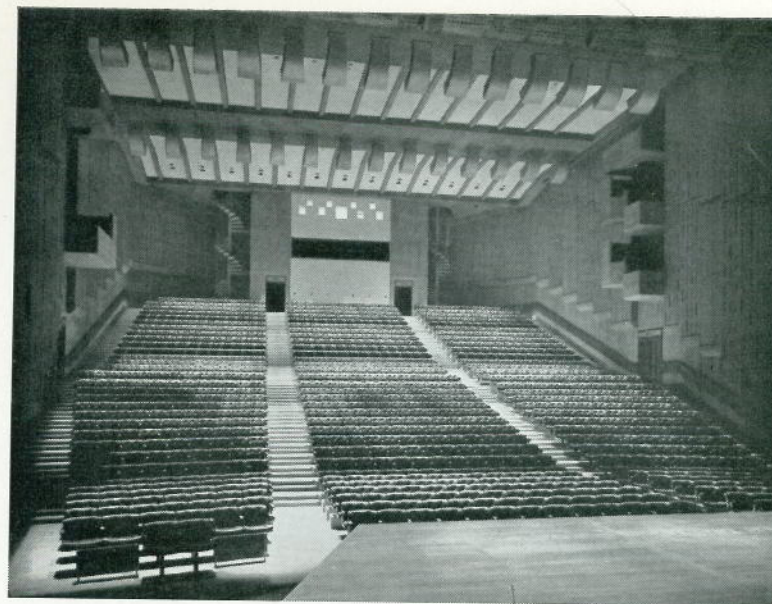
Queen Elizabeth Hall. View from platform showing ventilation scoops, television perches on side walls and control room with projection room above at rear.
