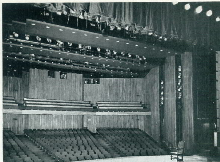
Abbey Theatre auditorium showing ceiling slots and FOH spots (see schedule of equipment on following page). The suggestion of benches in the balcony originates in the timber book ledges at the backs of the seats. (Below) Ceiling sections lowered to balcony level showing the raising gear and flexible feeds for lighting.
