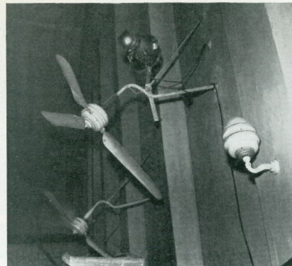
The fan bracket also provides the fixing for a Strand spot.
