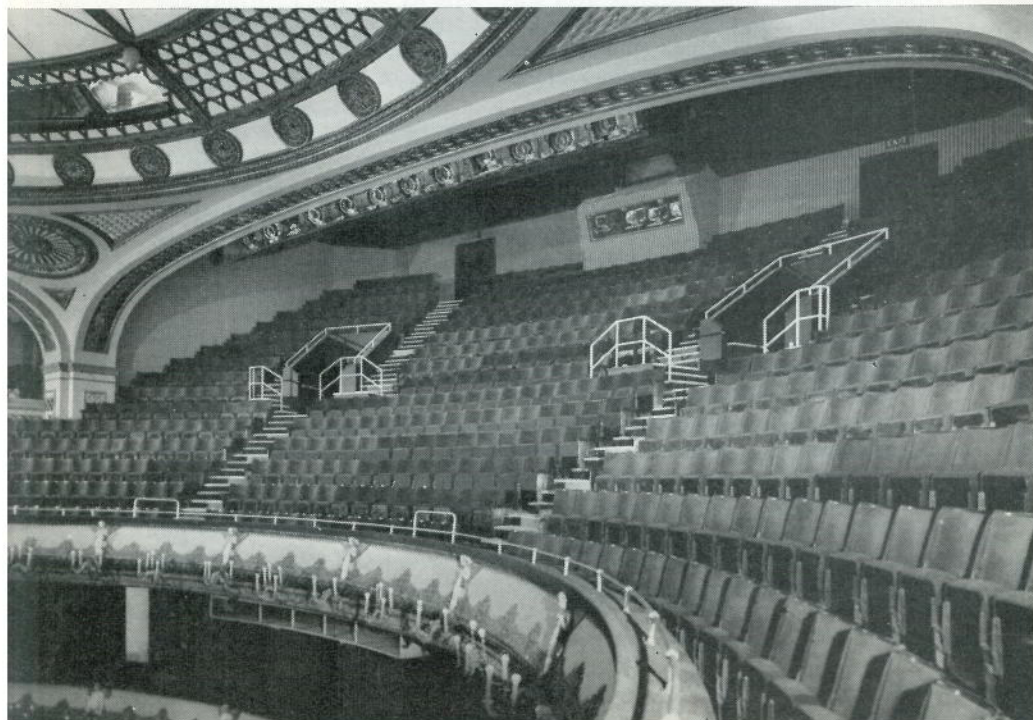
Fig. 2. Royal Opera House: new amphitheatre showing a dome follow spot aperture and FOH spotlight bridge. (Photo courtesy Bovis Ltd.)
