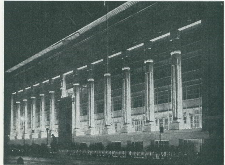
230 kW of G.E.C. floodlighting at the Black Cat factory in 1931 controlled by Mansell and Ogan automatic colour mixing dimmer.
