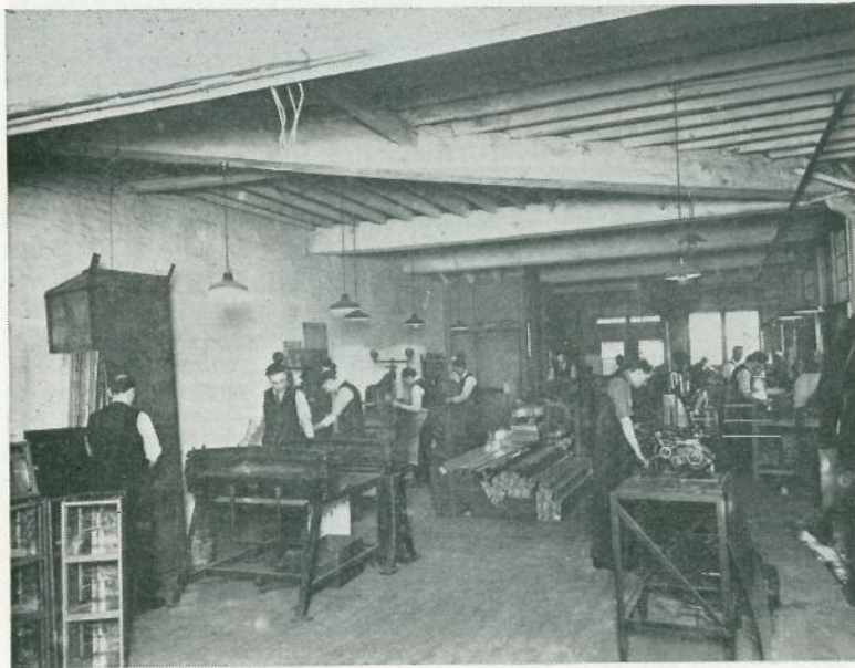
The Sheet Metal Shop, Floral Street, circa 1930. The 6 ft. Bender seen on the right is still in regular use, see p. 115.
