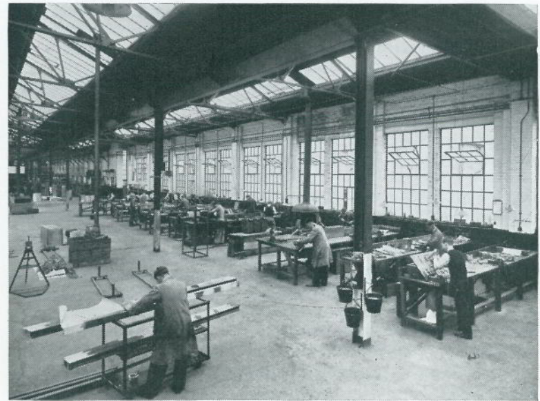
Workers thin on the ground. Part of the Ealing works shortly after the move in 1938.
