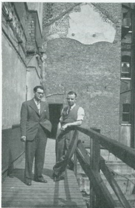
Jack Sheridan and Lorcan Bourke on temporary bridge over the ruins of the bombed demonstration theatre 1941.
