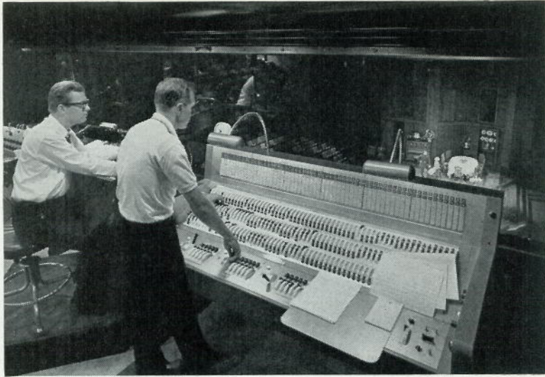
The Kliegl Lighting Control front of house with view of stage beyond; 60 dimmer channels, 3 presets. Push buttons on the vertical panel above the dimmer levers are for setting up groups within the presets.
