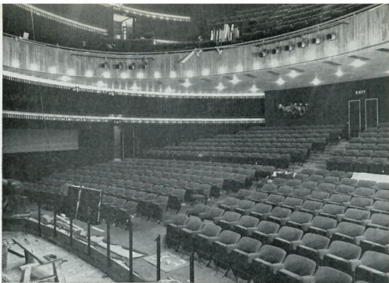
Fig. 6. View from apron stage entrance. Orchestra lift rises to stage level as two sections to provide a greater or lesser depth for this purpose. Orchestra wall supports foreground are removable. Lighting control box window is visible at rear of stalls.
