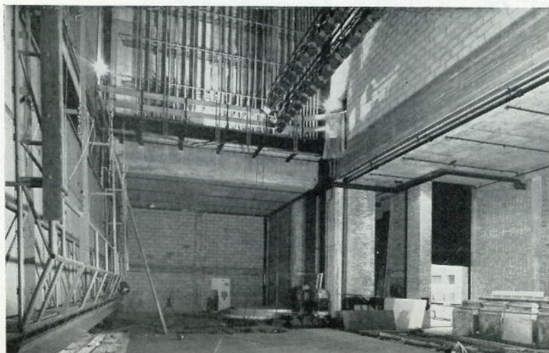
Fig. 7. Stage from P side wings with lighting bridge in the lowered position on the left. 26 ft. revolve can be seen in centre and cyclorama lighting bank top right. Partially raised black shutter shows paint frame room beyond.
