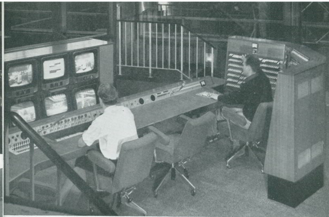
Fig. 6. Camera channels and 217 lighting circuits controlled by two men. (Photo by ABC TV).
