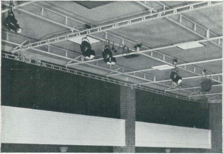
Fig. 7. Detail of grid and ceiling
