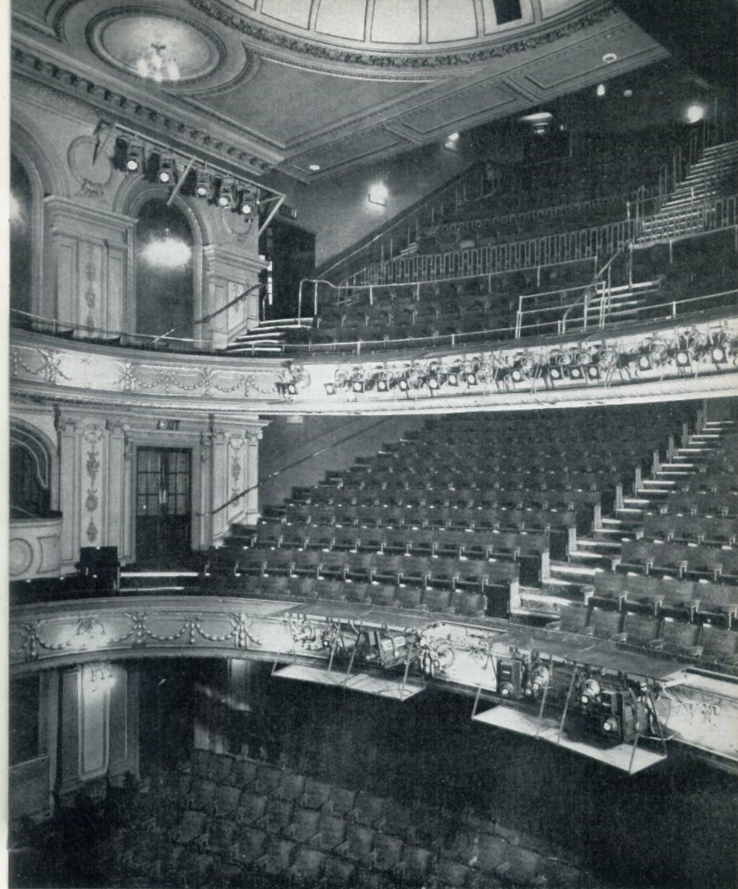
Auditorium, Aldwych Theatre, showing some of the new F.O.H. lighting. There are further positions adjacent to the stage boxes, altogether 33 dimmers are used for F.O.H. spots.
