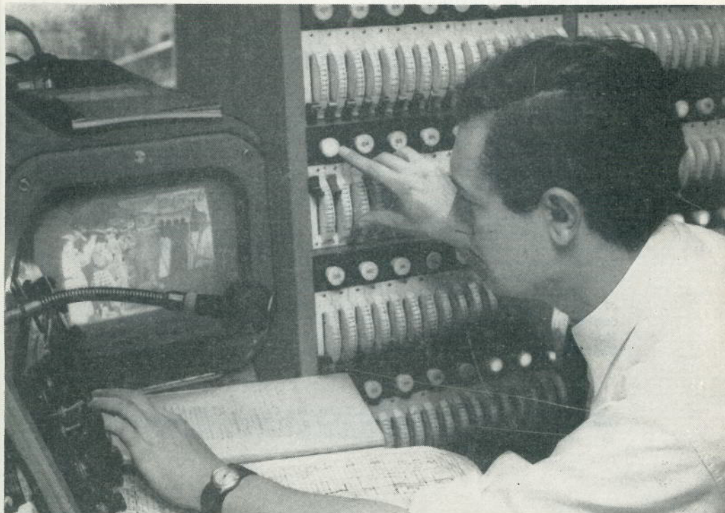
FIG. 3. B.B.C. Riverside 1. Lighting supervisor using monitor to set lighting. Photo by courtesy B.B.C.
