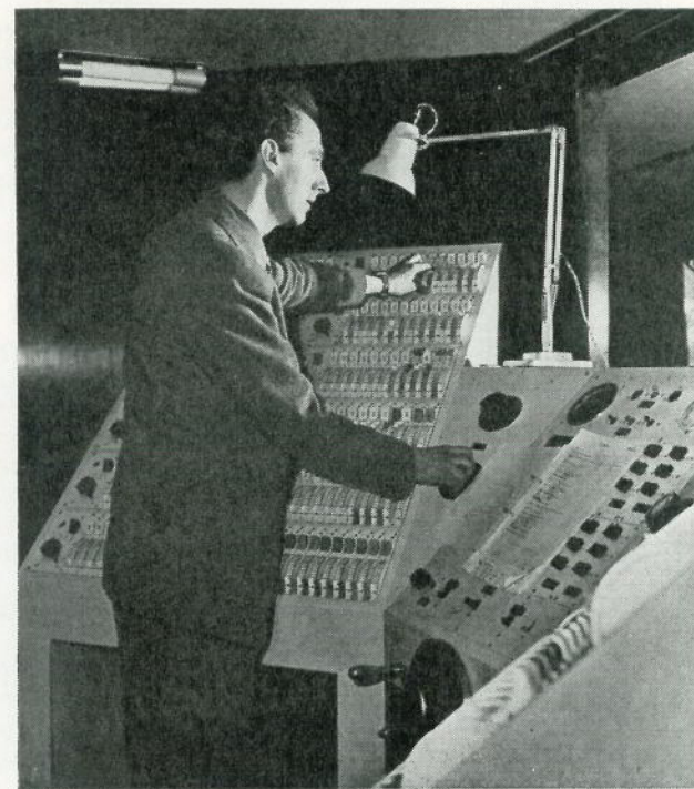
FIG. 3. Part of the Pre-set Switchboard situated in the front-of-house with an unobstructed view of the stage, at Shakespeare Memorial Theatre, Stratford-on-Avon, 1951.
