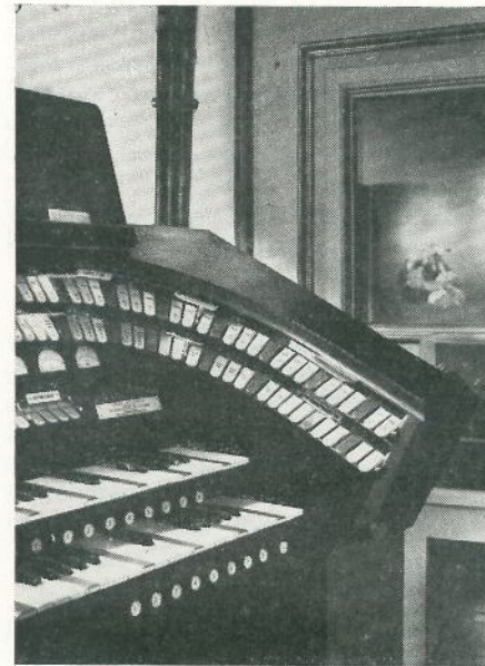
Fig. 1. The Strand Light Console at the Opera House, Ankara, is situated in a box in the front-of-house and the operator views the stage through the window at right.
