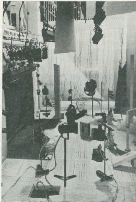
Fig. 3. General view of the stage and its equipment. The large spotlight with colour-wheel in the middle distance is ordinarily used for F.O.H. work. At the foot of its stand, a groundrow can be seen. The cyclorama is here shown flown, but the horizon floods which light it are visible just below the fly floor (top right). Note the match-box at stage centre.
