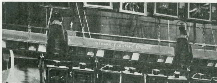
Fig. 3. German type Acting Area lanterns between 6-foot lengths of batten as installed at the Covent Garden Opera House in 1934.
