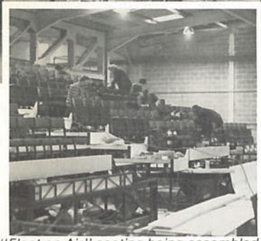
"Float on Air" seating being assembled.
