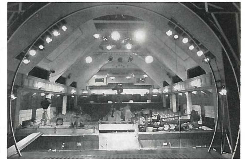
(Above) TV Production: FOH positions. Some 5 kW's are focused for audience shots and 2 kW for orchestra shots. 10 kW on camera rostrum used for lighting rings. At the back of the balcony, the lighting control box is to the right and sound control is to the left.
