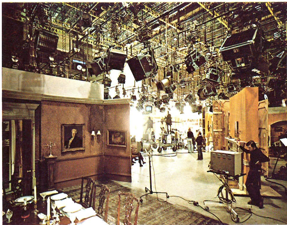
Studio 4 at Television Centre with a rehearsal in progress. Dual-Purpose 5½ kw lanterns hang from pantographs on motorised hoists above the setting area ready for immediate use. As far as possible the floor is kept clear for the cameras. Lights on sets not in use are switched off to save power.
