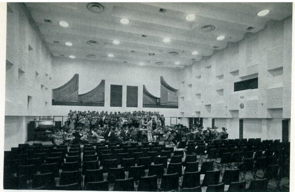
University of Cardiff and Monmouthshire. Department of Music, exterior below and the Rehearsal Hall above. Architect: Alex Gordon and Partners.
